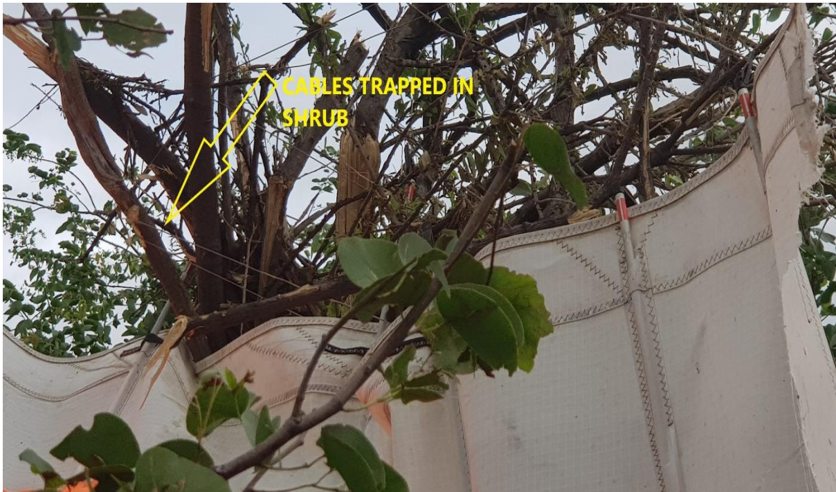
Fig. 3 Power Cable in Shrub
